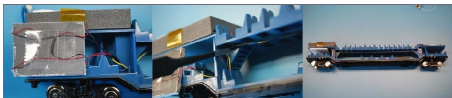
38. Lower-level front/rear lighting fixture installation and wire routing.
