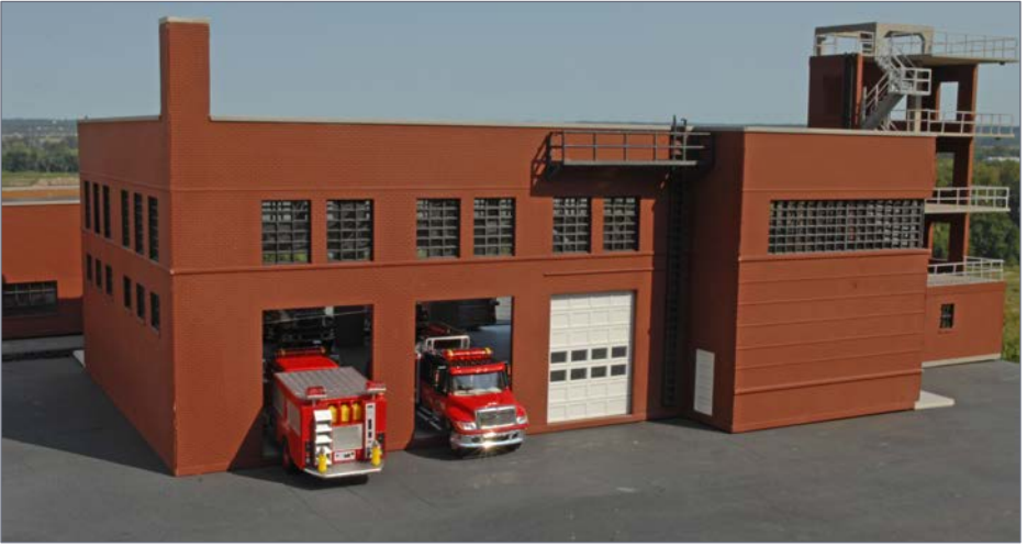
14. This shows the back side of the building with one of the bay doors installed in the down position.
