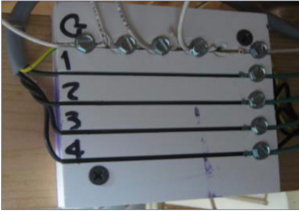
19. A five-slot block for five-conductor cable, clearly marked with a Sharpie.
