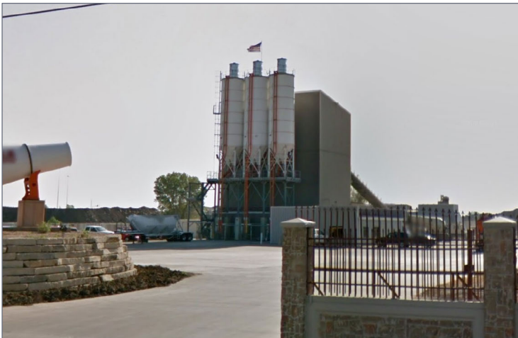
19. Andale Ready-Mix cement silos.
