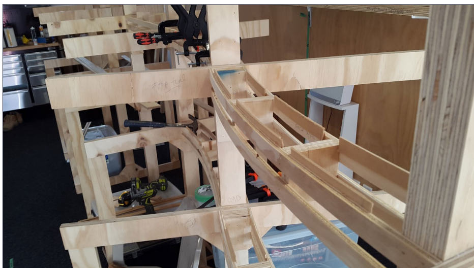
7. Setting the S curved section.
