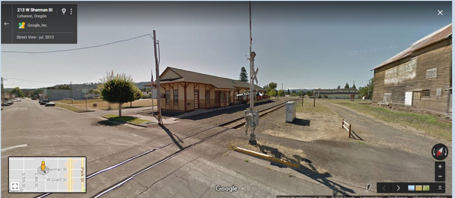
17. Santiam train station street view.
