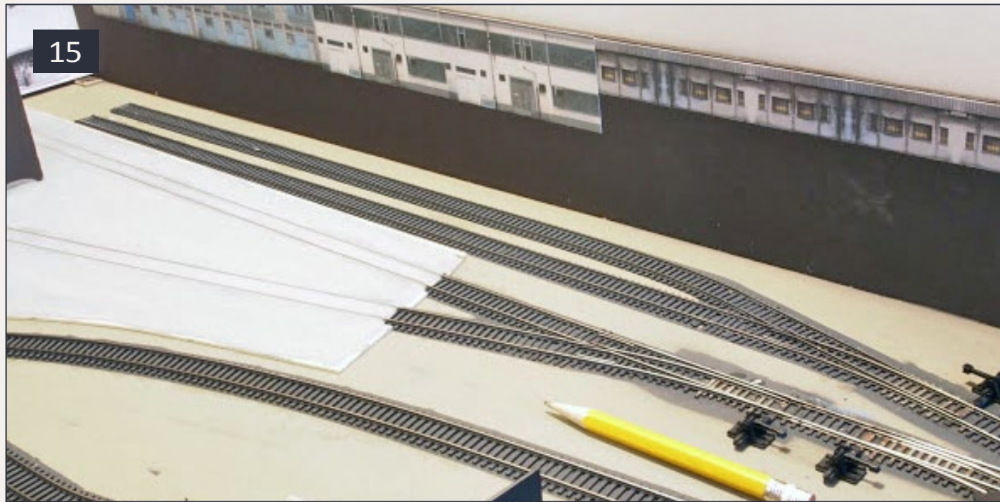
15: To prepare the cannery location, we affixed some cardstock background buildings that will show up behind it. On the upper left, you can also see the freight house concrete pad we poured using thinned and tinted light-weight spackle. When it dries we'll sand it smooth (so the ties still show through a little), and then weather it.
