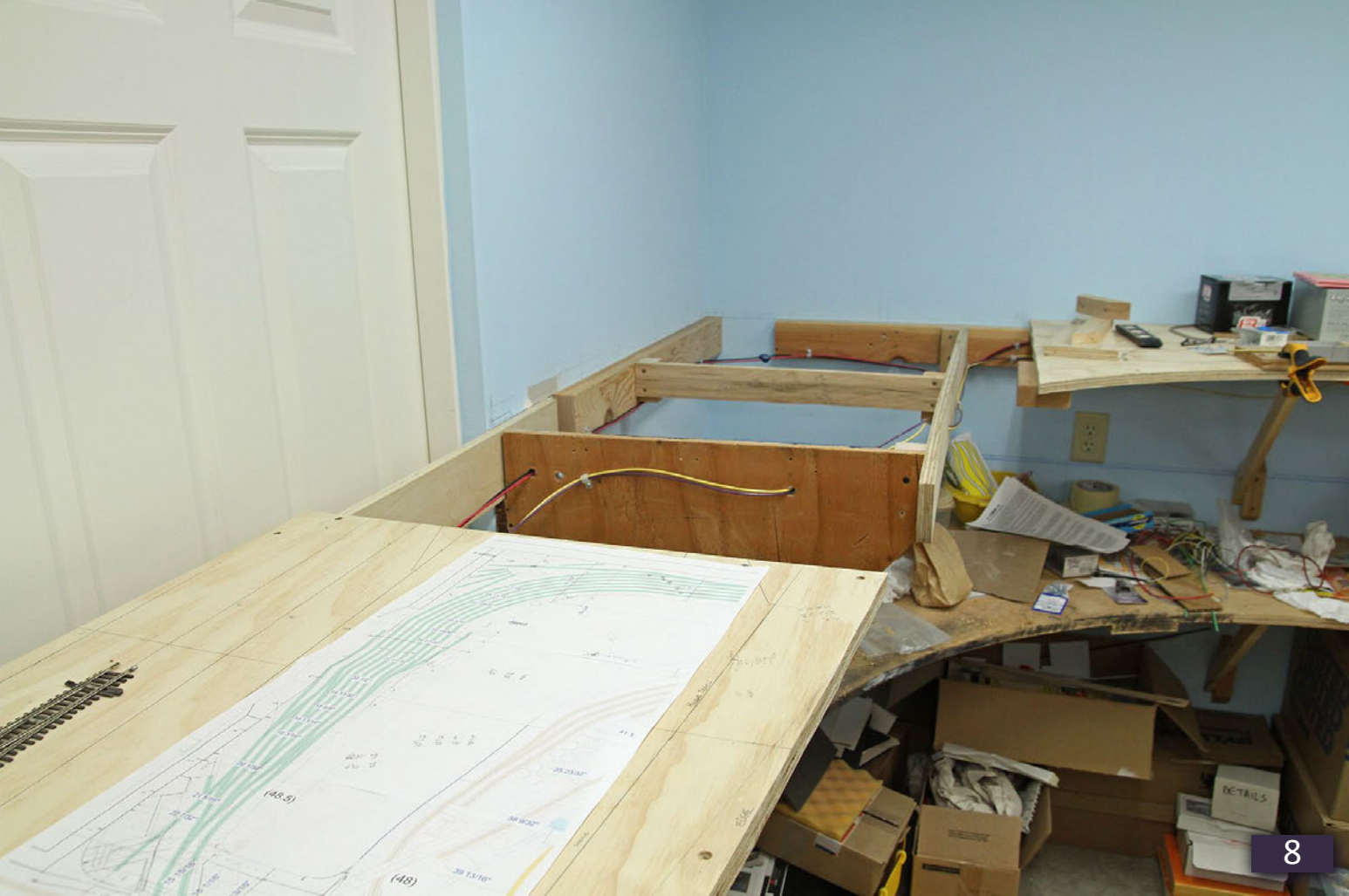
8, 9. South Jackson looking toward the turntable's corner. Most joists have been set in place and some wiring installed.
