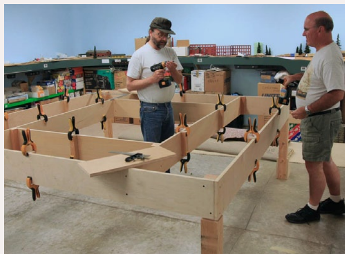
FIGURE 10: Construction of the helix table under-the-surface bracing.
