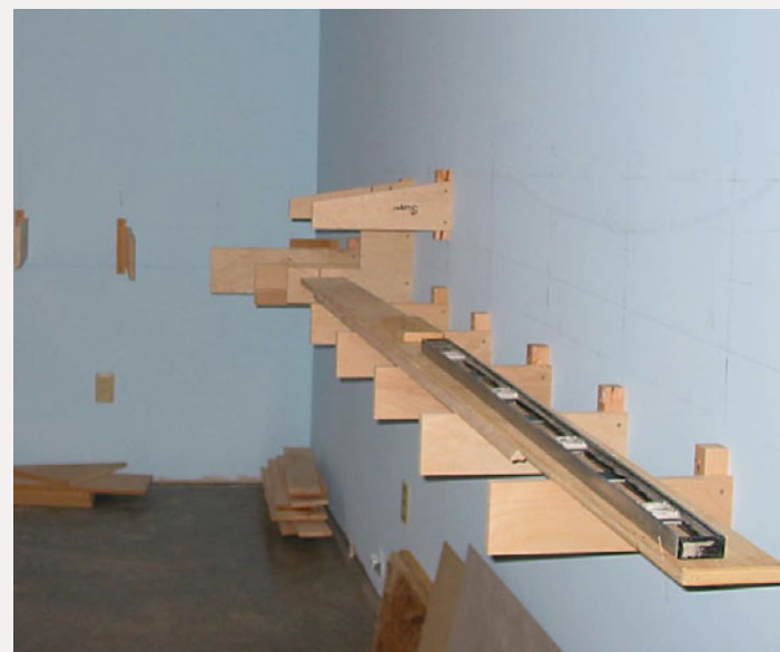
FIGURE 5: More joists and cleats.
