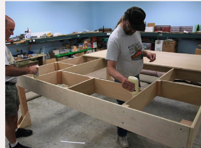
FIGURE 12: gluing the helix table top in place. Later on I'll cut out an area in the middle to provide pop-up access inside the helix.
