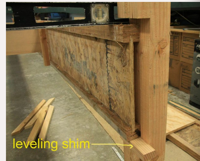
FIGURE 15: Shimming the engineered joists to level them.
