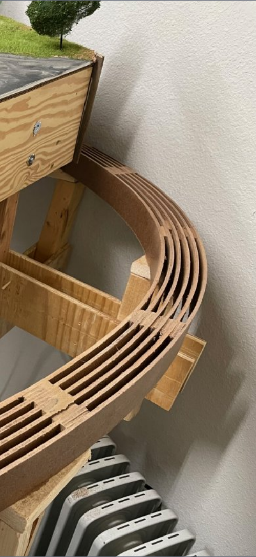
19. The “hidden ramp to staging” under construction.
