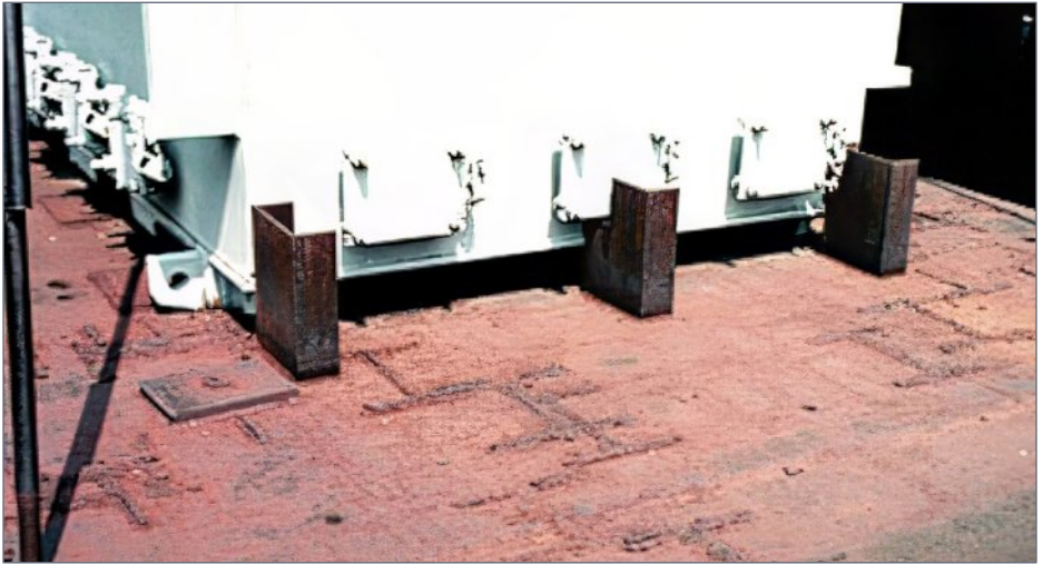
3. Prototype steel blocking welding remnants.
