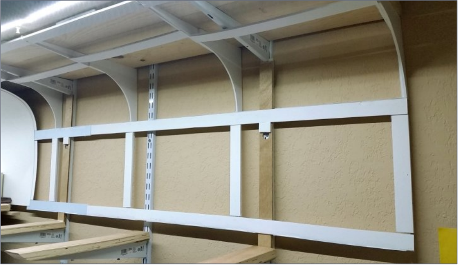
33. I built a framework for matte board to permit a curved backdrop, since the matte board is thin enough to bend.
