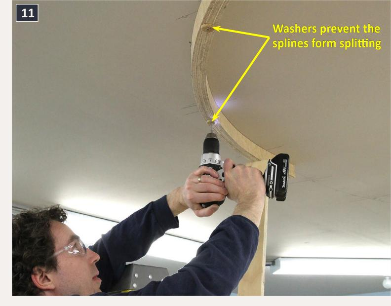
11. Mounting the Masonite spline on the ceiling with 3-1/2" deck screws is work! Note the washers used to prevent the screw heads from splitting the splines. I made my own washers from Masonite with a 1" hole cutter, but metal washers would also work. We needed to coax the spline just a tad to keep it lined up with the ceiling marks.
