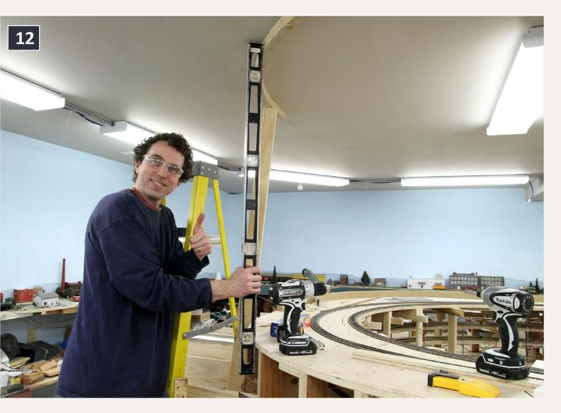
12. We double-checked the ceiling cleat's alignment with the benchwork below. To our relief, it was spot on!
