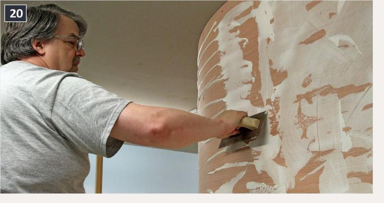
20. I ran a lot of construction adhesive beads onto the backdrop, then spread it around with a notched trowel.
