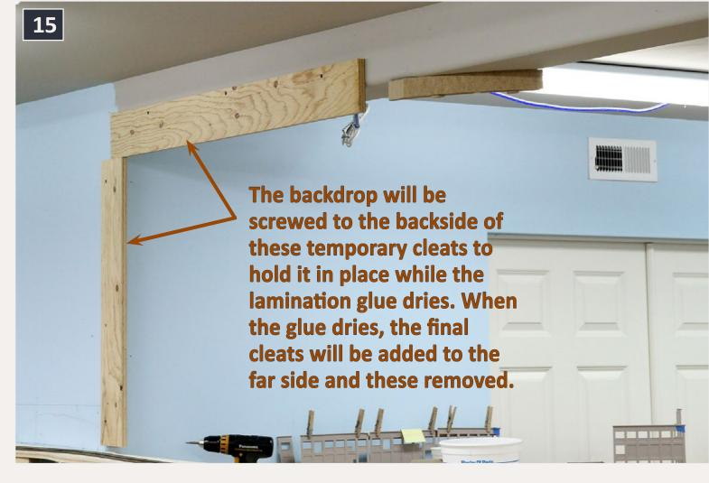
15. The first piece of backdrop has to be flush with the wall on this side. I temporarily screwed a couple of ¾" plywood guides to the wall. The backdrop will be on the far side of these and screwed to them. Once the glue set, I removed the screws holding the backdrop to the temporary mounts, screwed cleats in place on the South Jackson (far) side [25], and then removed the temporary 3/4" plywood guides. Once spackled, the resultant joint is almost perfectly flush.
