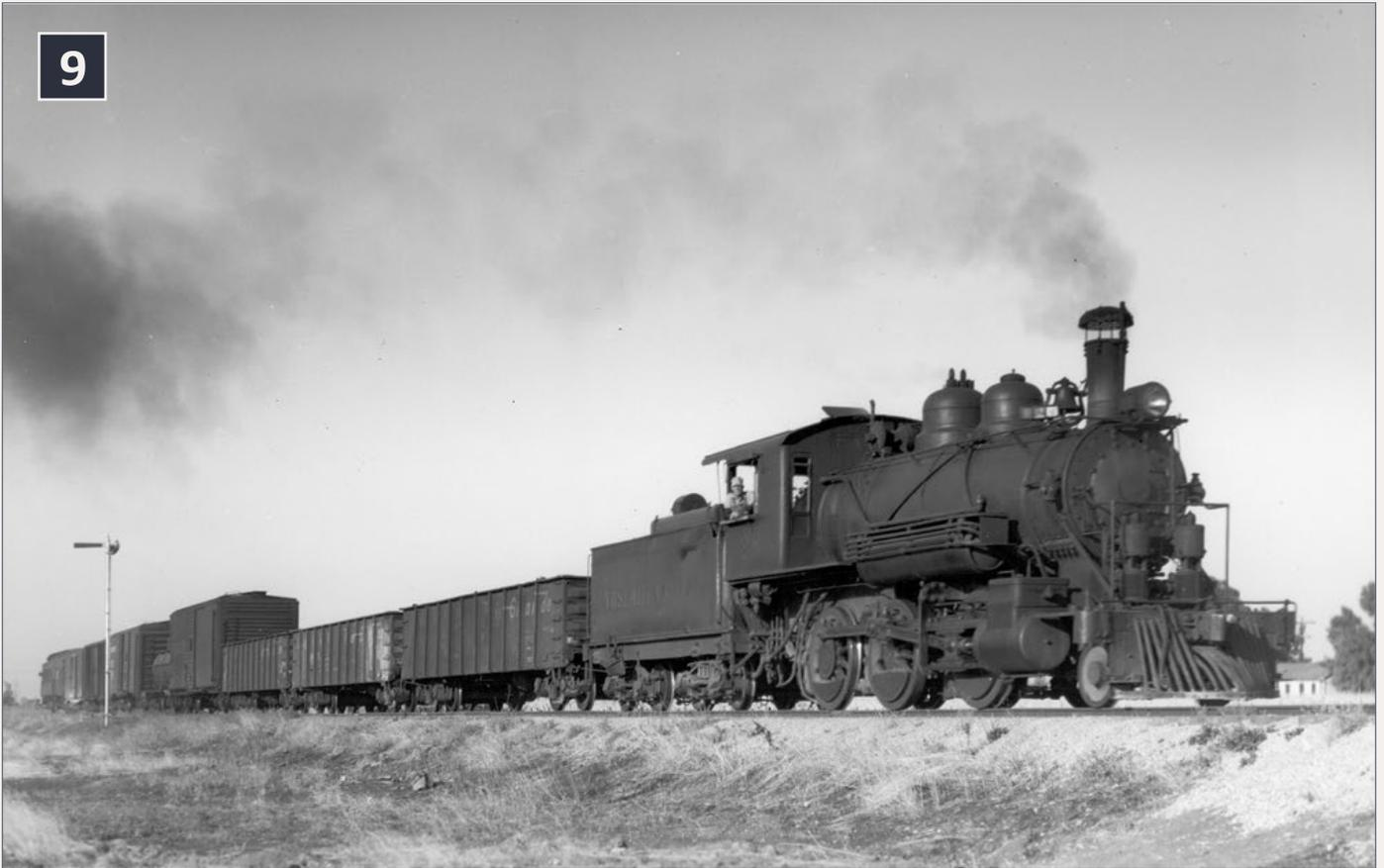
**9: There are no known photos of local freights on the YV while they were running as extras. However, this photo of a mixed train leaving Merced sometime after June 1943 shows what might have been a typical consist in those days. The engine has just passed the semaphore for the AT&SF interlocking plant (Fred Stoes photo).**
