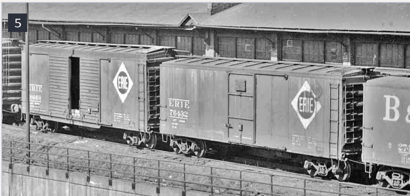
5. Erie 76432 at Akron, OH in April 1959. Note that the original door has been replaced with a Superior door. The car has been repainted at some point in time, most likely when the sides of the car were repaired. The small diamond has been replaced with the larger Erie diamond, however the small Erie Diamond can be seen ghosting through the new paint. (Authors collection and used with permission of George Elwood Fallen Flag Railroad Photos.)
