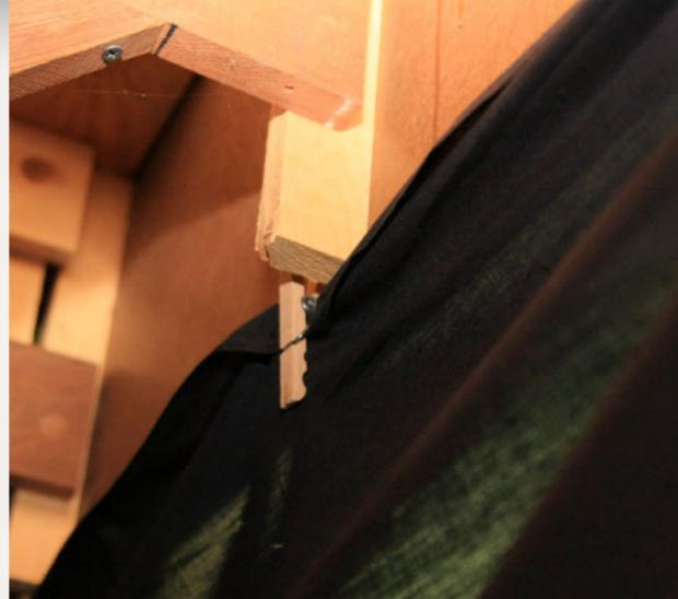
Figure 5: Spring-loaded clothes pins make curtain installation and removal easy.
